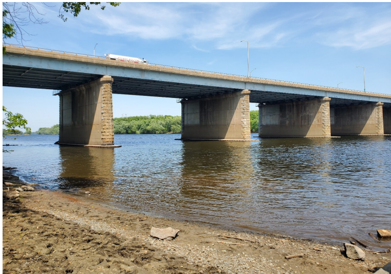
Site of DV01 looking upriver from boat ramp
