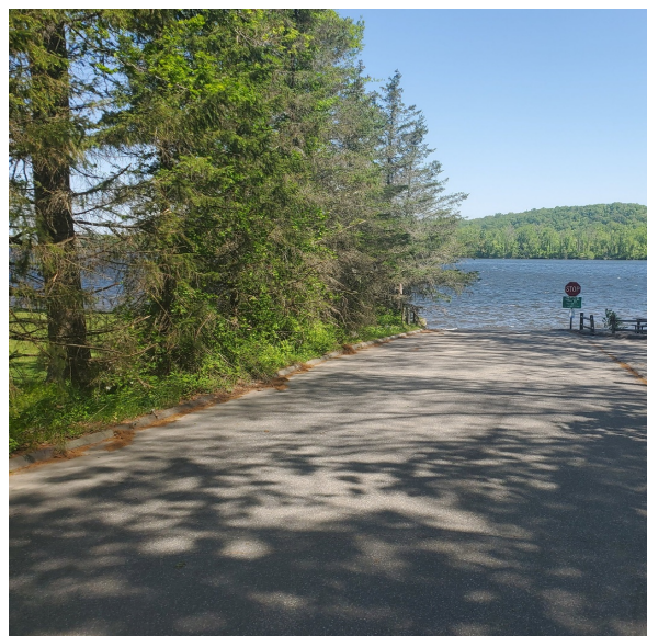
Parkers Point Boat Ramp parking/staging area looking northeast toward boat ramp.
