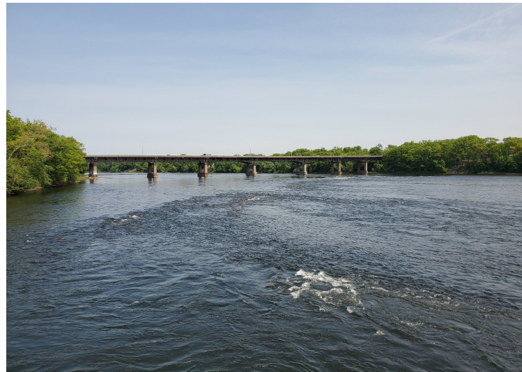
Looking upriver from Windsor Locks canal head. Site of DF01 and parking/staging area on left
