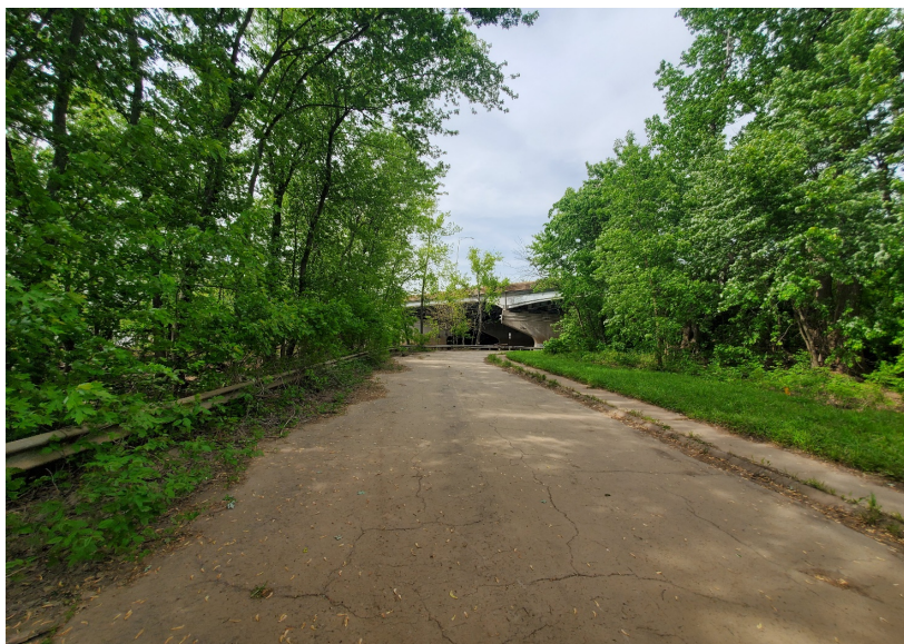
Access road to Cove entrance canal looking north from Cove Park parking/staging area. CT River to right of photo.
