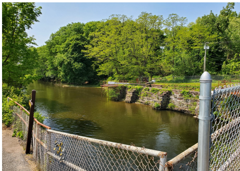
Looking south from Windsor locks canal head to site of DV02 inside canal
