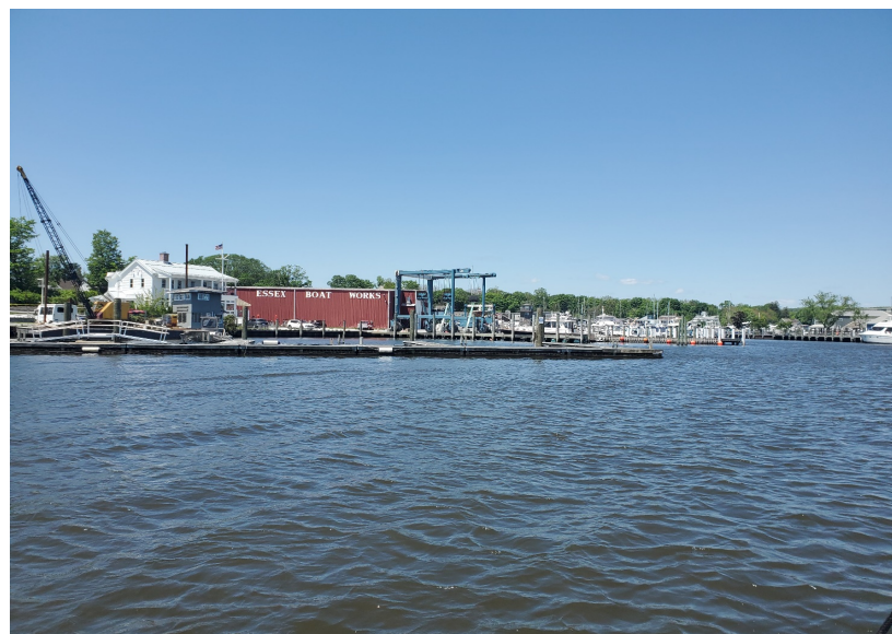
Entrance to Safe Harbor/Middle Cove (right) and site of EX01d looking west.
