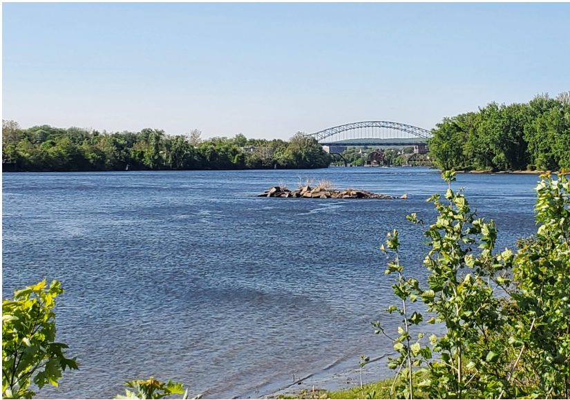
View looking south/downriver toward Mattabessett River (on right) and site of EX02 and flood tide DV01alt strategy.
