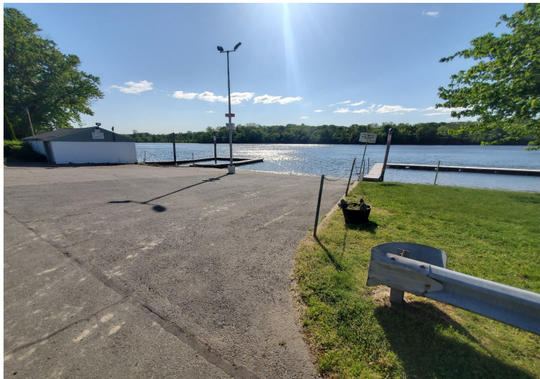
Cromwell Outboard Association boat ramp looking east/upriver (left) toward site of ebb tide DV01 strategy.
